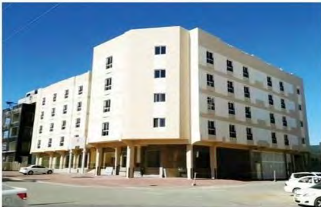
Residential Commercial Building, G+4, Bait Fatma – USD 3.12 Million
