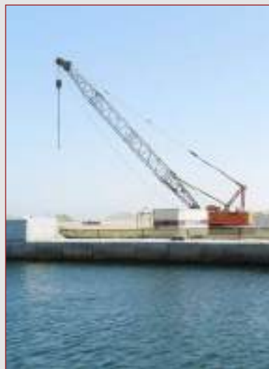
◀ QUAY WALL UNITS INSTALLATION
