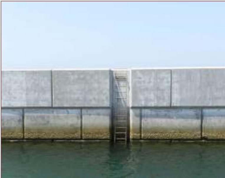
▲ QUAY WALL AND CAPPING BEAM
