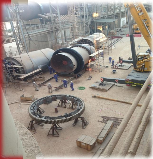
Replacement of Kiln shell , Girth gear , Tyre, Rollers, Cowl shell for LINE# 2 M/s FLSMIDTH , OMAN CEMENT CO.
