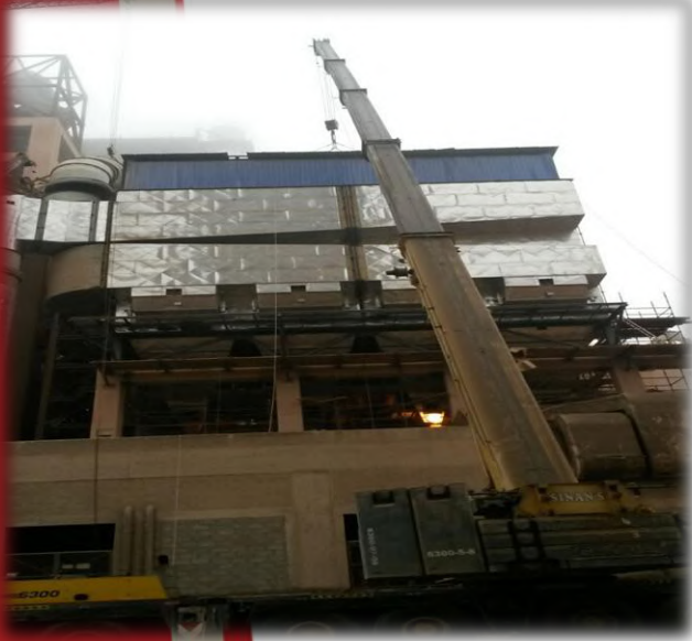
Dismantling of LINE#3 Existing ESP and Conversion to New Bag filter for M/s CTP , Italy , RAYSUT CEMENT CO.SAOG
