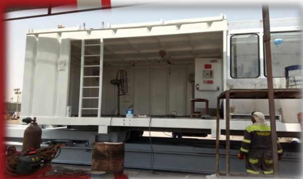
Maintenance works of Dog house for M/s ABRAJ ENERGY SERVICES
