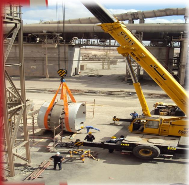
Replacement of Kiln shell , Girth gear , Tyre, Rollers, Cowl shell for LINE# 2 M/s FLSMIDTH , OMAN CEMENT CO.
